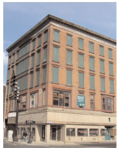
The Downtown North Historic Rehabilitation project will include over 500 residential units (Phases III and IV) in three rehabilitated historic buildings and one new 14-story tower, as well as 100,000 sf of retail and commercial space.
